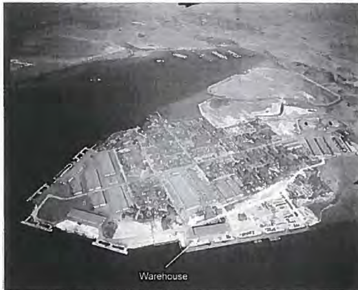
Enclosure 17. Overview of the Pearl City Peninsula showing the Supply Center Provisions Annex warehouse in 1948, view to Northwest.
